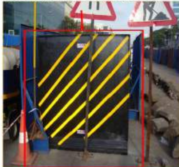
Barricading Boards for nosing
