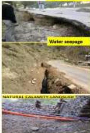
Road Collapsed
