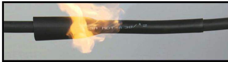
Heat Shrink Sleeve and Aluminum foil is used to seal the joint closure
