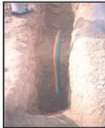
Bending Radius Not Maintained during Laying
