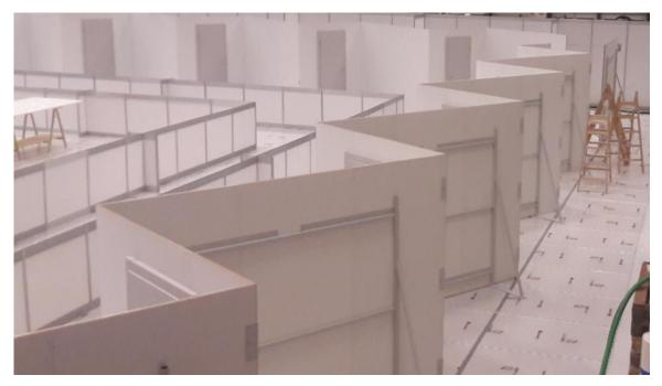
Sample workshop layout: Side with the door: 2.00 m x 2.50 m, Side with no door: 4.00 m x 2.50 m
